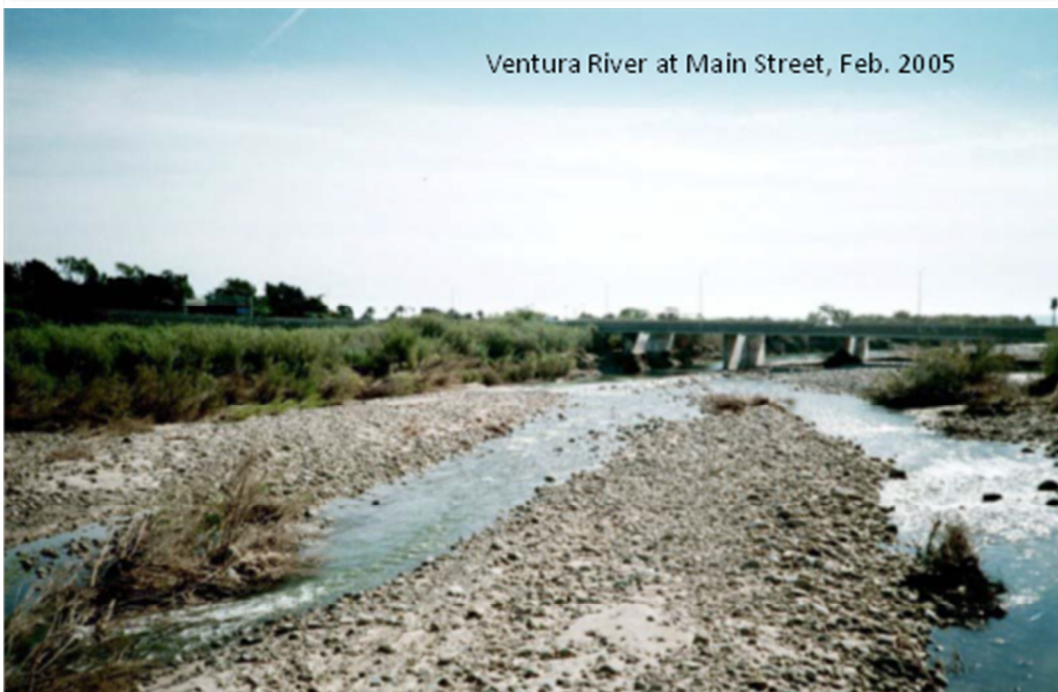
Figure 2-17 Main Street Bridge 2005
